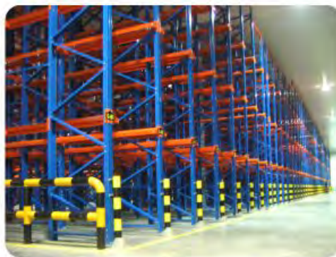
Cold Storage -32°C
