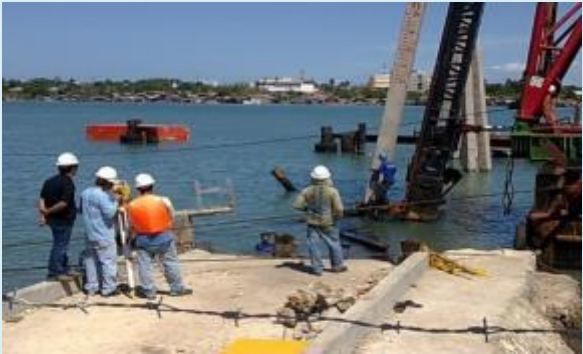
Petron Corporation Mandaue Terminal Proj. Determining exact pile location
