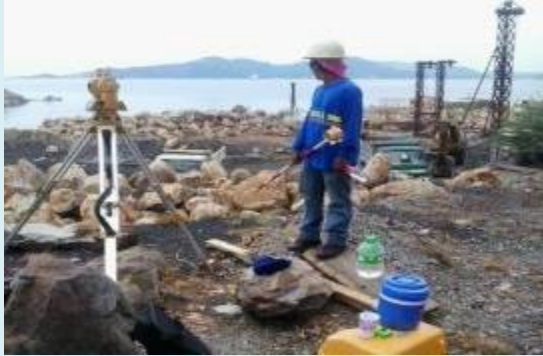
SMC Shipping & Lighterage Corp. Geotechnical Investigation Establishment of Grid Line
