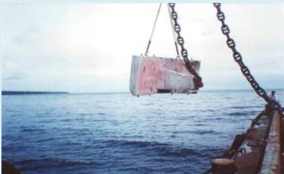
5-Ton Concrete Anchor ready for deployment underwater
