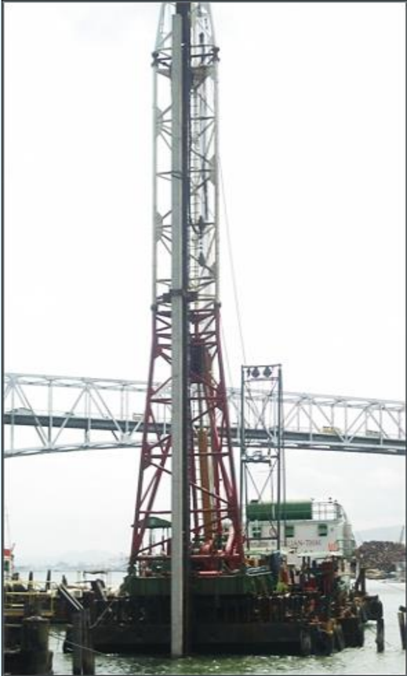
Pile Barge #2 holding a concrete pile ready for driving
