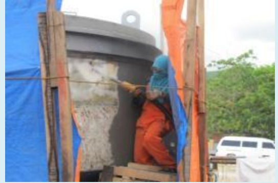
PHILIPPINE MINING SERVICES CORP. Sandblasting of Mooring Buoy
