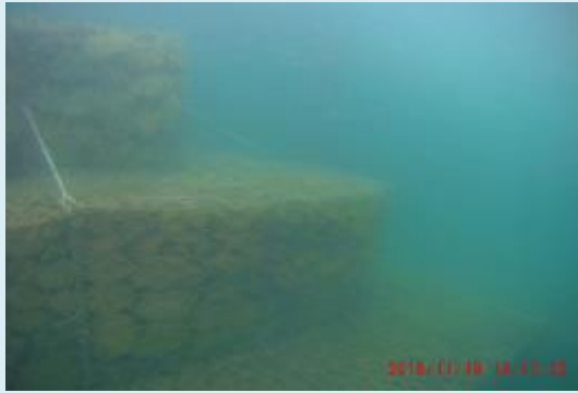
SOUTHERN PACIFIC INCORPORATION Installed Boulders/Gabion PROPOSED GABION SILT INTRUSION PROTECTION
