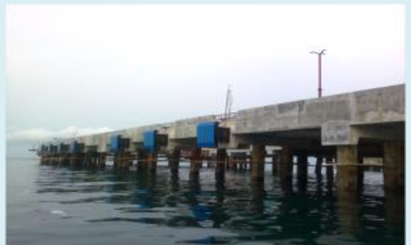
Completion of the Domestic Loading Area at the Orca Nitrates Pier, Negros Oriental
