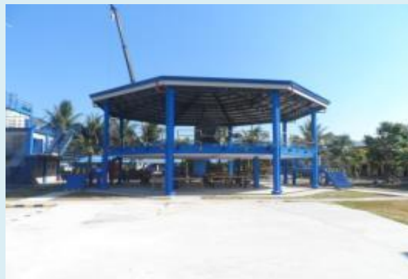
CONSOLIDATED TRAINING SYSTEM, INC. Completed Construction of Helideck at Tanza, Cavite
