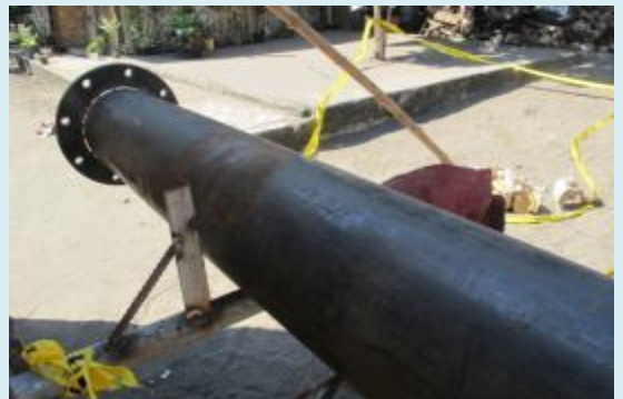
PETRON CORPORATION Fabrication of Stainless Steel Ladder and 8"Ø Pipe for the Repair of Pier and 8"Ø Riser Pipe
