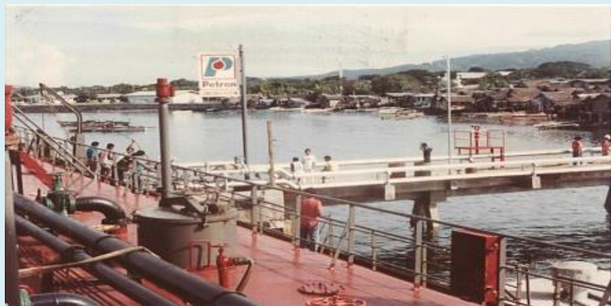
1 st fuel receiving at the newly constructed Petron Zamboanga Depot
