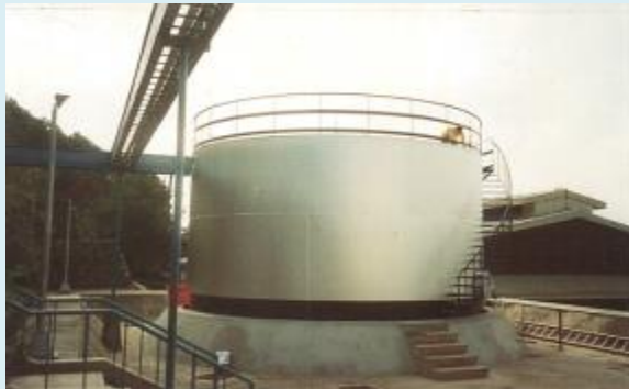
Completed Unit of the Fuel Tank Storage at Petron Zambonga Depot
