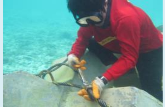
SEVEN SEAS RESORT & LEISURE, INC. Underwater Securing of Steel Cable on Concrete X-Block for Wave Breaker
