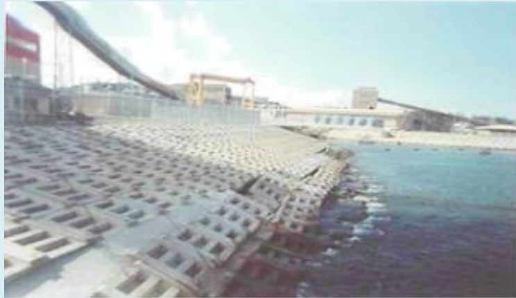
Armour Rocks and Gabions Laying Project
