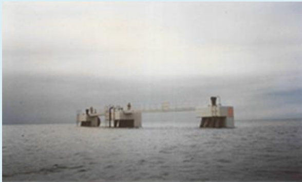
Completed Berthing & Receiving Facility with Underwater Pipelines
