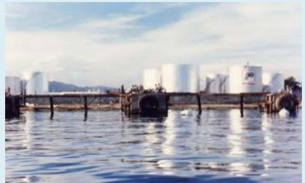
Front view of the Petron Corporation Zamboanga Depot pier facility
