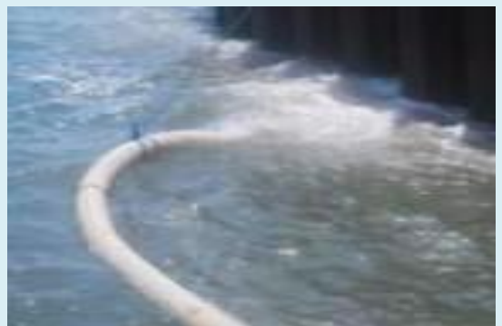
STA. ELENA CONSTRUCTION AND DEVELOPMENT CORPORATION Water jetting and airlifting for the Underwater Installation of GRP Pipes at Batangas City
