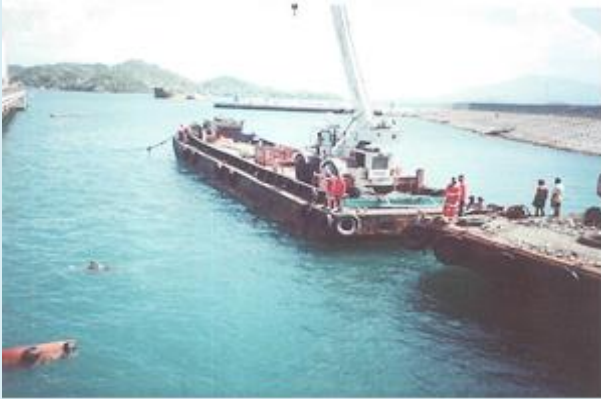
Armour Rocks Hauling and Installation at Team Energy Sual, Pangasinan
