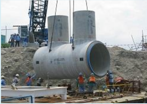
Naphtha Intake Structure Construction
