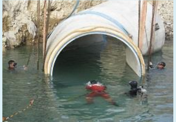
Naphtha Plant Intake Pipe Laying
