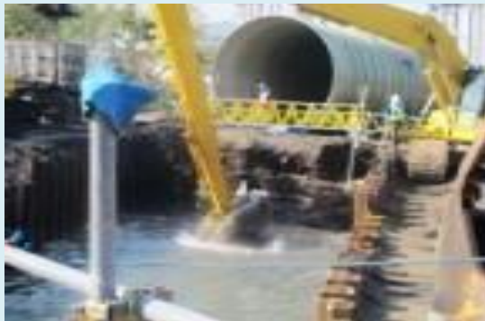
STA. ELENA CONSTRUCTION AND DEVELOPMENT CORPORATION Dredging work prior to GRP pipe laying for the Underwater Installation of GRP Pipes at Batangas City
