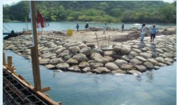
Interconnection to the Pier Deck
