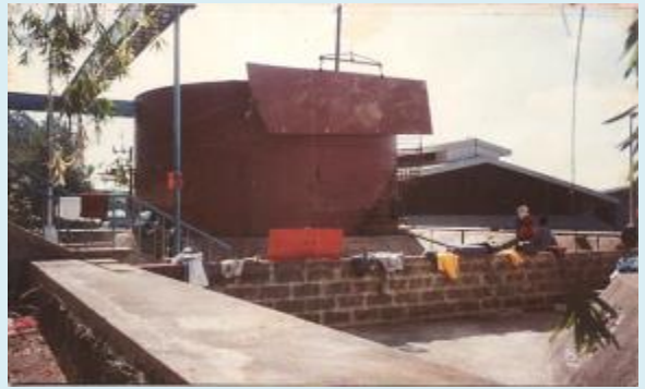
Fuel Tank Storage Construction at Petron Zamboanga
