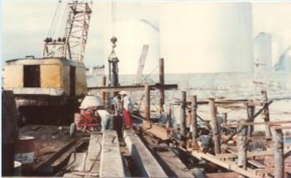
Construction of the Petron Corporation Zamboanga Depot
