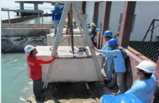
CEBU PRIVATE POWER CORPORATION Positioning of Completed Blocks for the Seawall Repair Using Concrete Blocks
