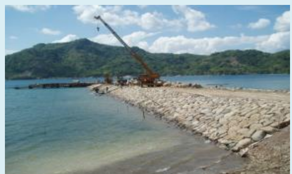
View of the construction of SM-Hamilo Ferry Terminal at Nasugbu, Batangas
