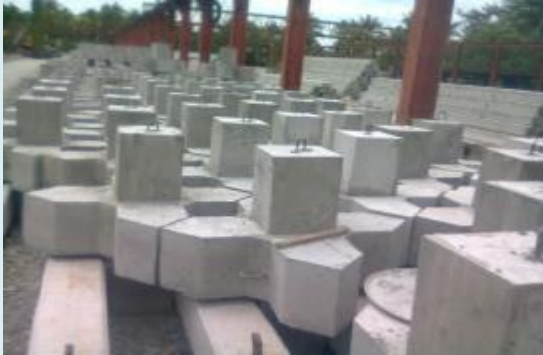
SEVEN SEAS RESORT & LEISURE, INC. Fabricated Concrete X-Block for Wave Breaker
