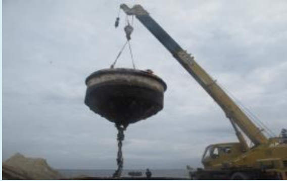
PHILIPPINE MINING SERVICES CORP. Retrieved Mooring Buoy for Rehabilitation
