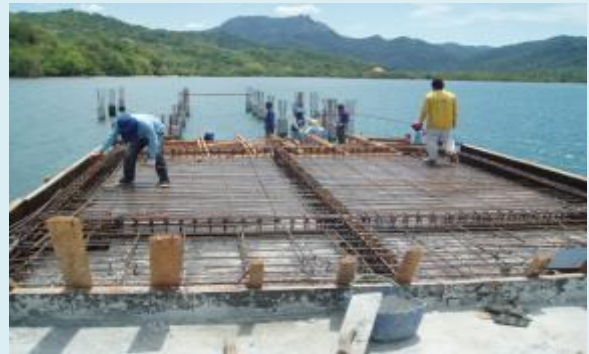
Steelworks and Formworks at the Pier Deck
