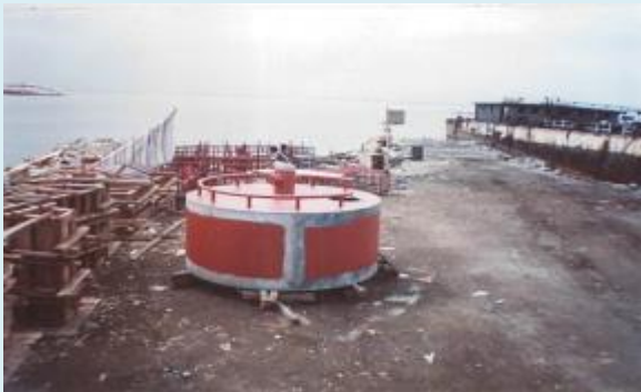
Application of marine coating system in preparation for top coat
