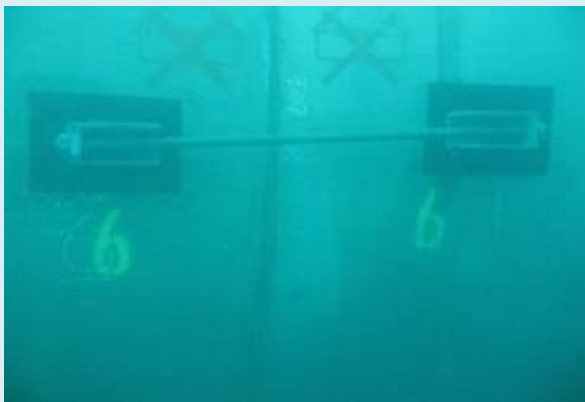
Naphtha Plant Intake Pipe Laying
