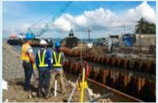
STA. ELENA CONSTRUCTION AND DEVELOPMENT CORPORATION Surveyors and divers conducted pipe elevation and alignment for the Underwater Installation of GRP Pipes at Batangas City
