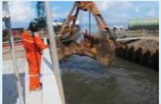
STA. ELENA CONSTRUCTION AND DEVELOPMENT CORPORATION Dredging work prior to GRP pipe laying for the Underwater Installation of GRP Pipes at Batangas City
