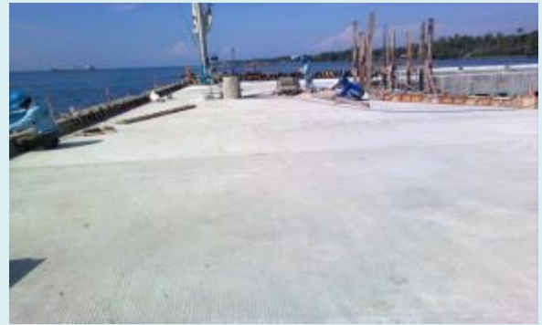
Pier Deck Completion
