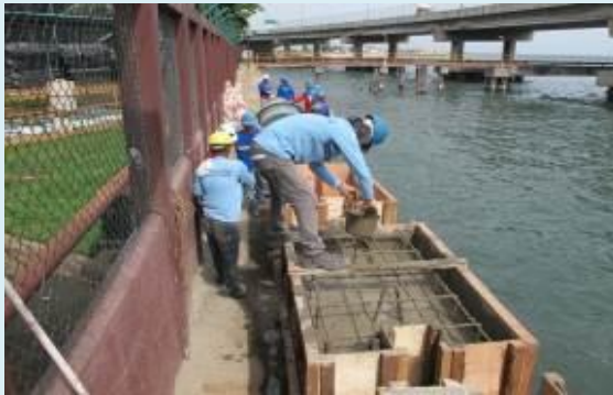
CEBU PRIVATE POWER CORPORATION Fabrication of Forms & Rebars and Concrete Pouring for the Seawall Repair Using Concrete Blocks
