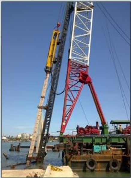
Concrete Pile driving
