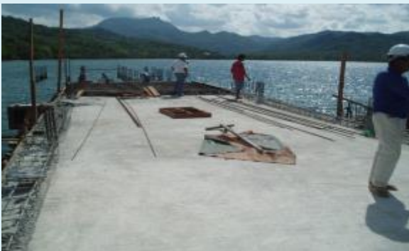
Concreting work activities on PierDeck
