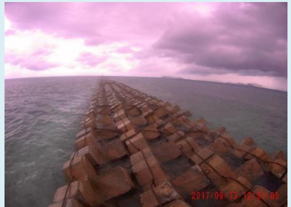
Pamalican Resorts, Inc. 50 Meters X-Blocks Extension Installed at Cuyo, Palawan
