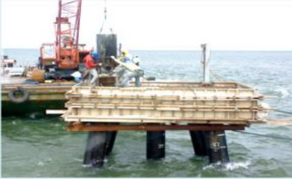
Concrete pouring of Newly Constructed Breasting Dolphin at Oilink Int'l., Bataan
