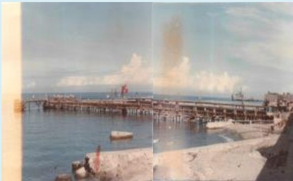
Near completion of the Petron Corporation Pier facility
