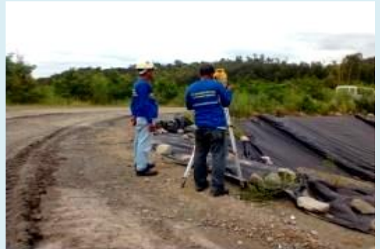
SMC Shipping & Lighterage Corp. Geotechnical Investigation Establishment of Grid Line
