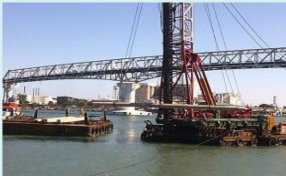
Petron Corporation Mandaue Terminal Proj. Pile Barge #2 setting from service barge
