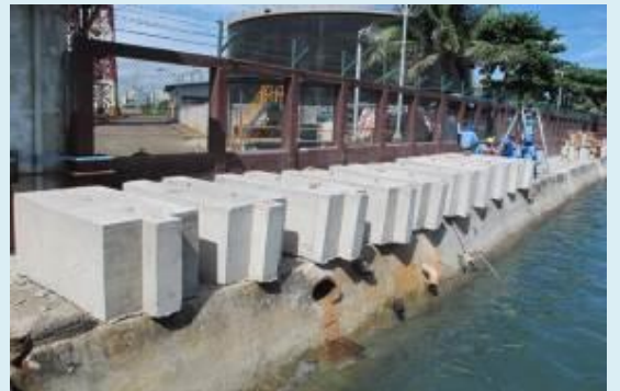
CEBU PRIVATE POWER CORPORATION Positioning of Completed Blocks for the Seawall Repair Using Concrete Blocks
