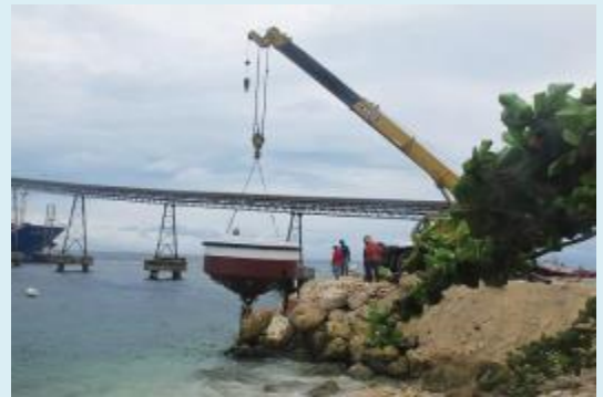
PHILIPPINE MINING SERVICES CORP. Launching of Mooring Buoy
