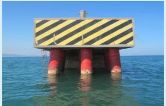
PETRON CORPORATION Above and underwater installation anti-corrosion paste, marine tape & FRP for the Repair of Pier and 8"Ø Riser Pipe
