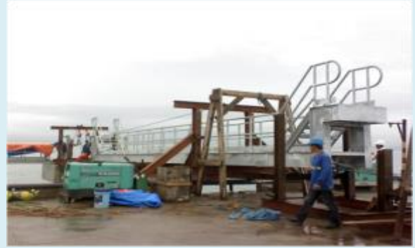
Construction of 1 of 3 Catwalks for the Breasting Dolphin Interconnection
