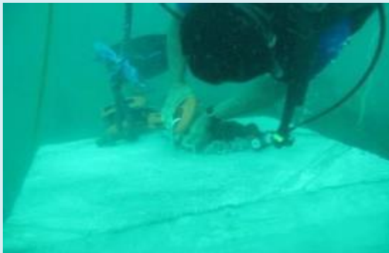
SIEMENS POWER OPERATIONS, INC. Underwater installation of concrete sinker to the drop point for the Supply and Installation of Marker Buoy Accessories at Batangas City
