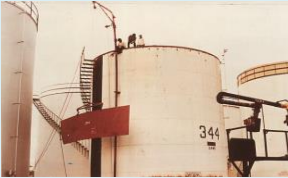
Fuel Tank Storage at Petron Zambonaga
