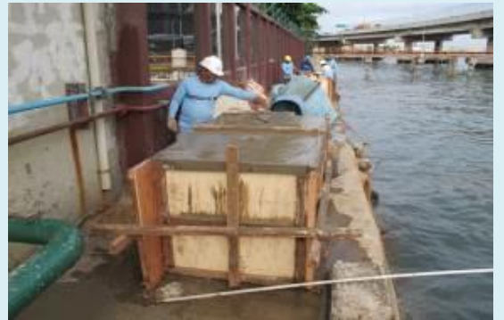
CEBU PRIVATE POWER CORPORATION Fabrication of Forms & Rebars and Concrete Pouring for the Seawall Repair Using Concrete Blocks
