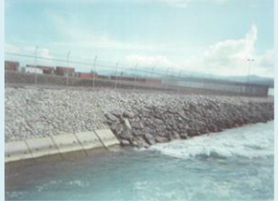
Armour Rocks and Gabions Laying Project
