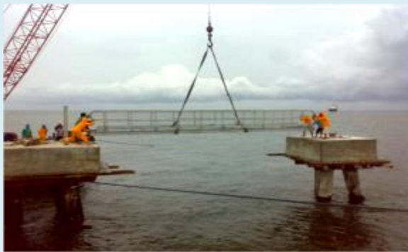
Installation of Catwalk for Breasting Dolphin
