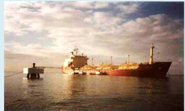
1 st product receiving on the newly commissioned Receiving Facility
