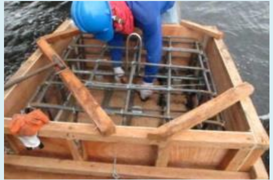
SIEMENS POWER OPERATIONS, INC. Fabrication of forms and rebars for the Supply and Installation of Marker Buoy Accessories at Batangas City
