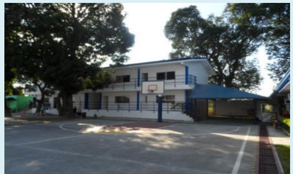
CONSOLIDATED TRAINING SYSTEM, INC. Completed Construction of Building for Two (2) Storey Classroom at Tanza, Cavite
