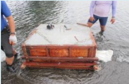
SIEMENS POWER OPERATIONS, INC. Concrete pouring and stripping of form for the Supply and Installation of Marker Buoy Accessories at Batangas City
