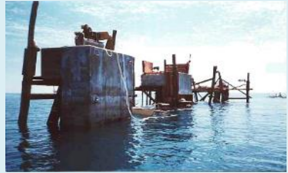
Berthing & Receiving Facilities Construction at Prycegases Inc.
