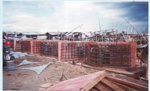
Concrete Anchors for the 4-point Mooring System
