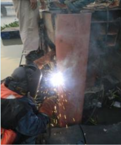
PDSI - Petron Corporation Installation of Steel Fender Support at Pandacan, Manila
