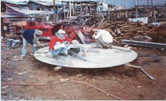
On-site construction of Mooring Buoys
