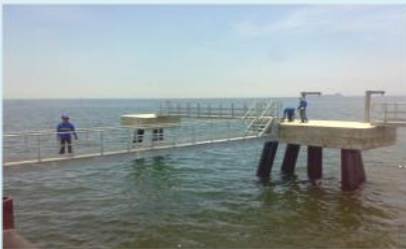
Interconnected Breasting Dolphin Facility construction completed
