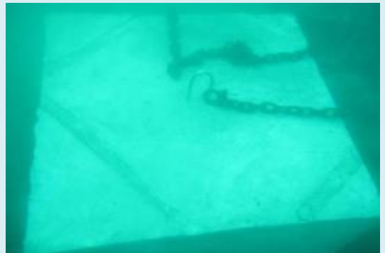
SIEMENS POWER OPERATIONS, INC. Underwater installation of concrete sinker to the drop point for the Supply and Installation of Marker Buoy Accessories at Batangas City
