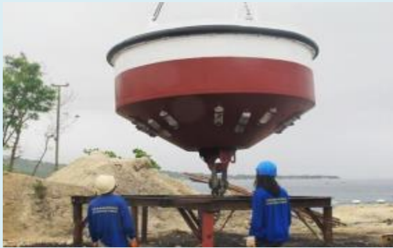
PHILIPPINE MINING SERVICES CORP. Mooring Buoy after Rehabilitation
