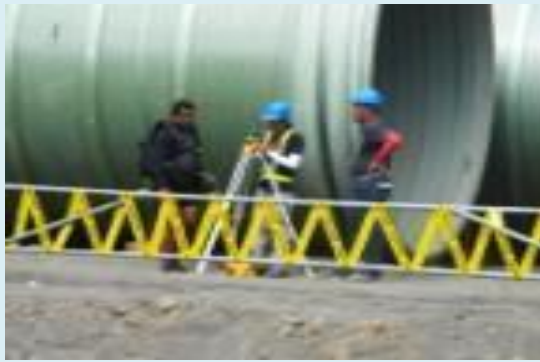
STA. ELENA CONSTRUCTION AND DEVELOPMENT CORPORATION Surveyors and divers conducted pipe elevation and alignment for the Underwater Installation of GRP Pipes at Batangas City
