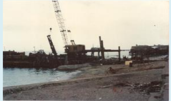
Offshore pile driving at the Petron Corporation Depot
