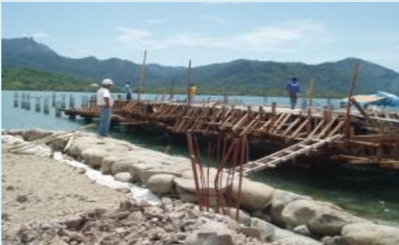
SM-Hamilo Ferry Terminal Pier Deck
