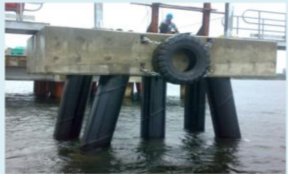
Completed Breasting Dolphin construction
