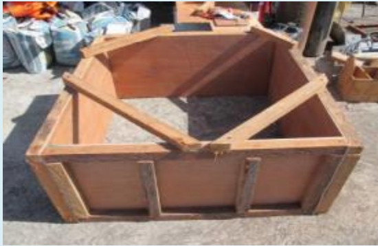
SIEMENS POWER OPERATIONS, INC. Fabrication of forms and rebars for the Supply and Installation of Marker Buoy Accessories at Batangas City
