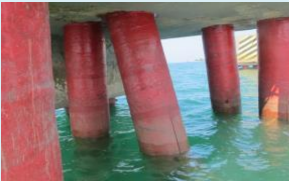
PETRON CORPORATION Above and underwater installation anti-corrosion paste, marine tape & FRP for the Repair of Pier and 8"Ø Riser Pipe
