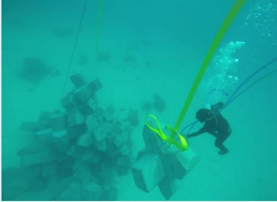
Pamalican Resorts, Inc. Underwater Retrieval of X-Blocks from the Drop-off Point at Cuyo, Palawan
