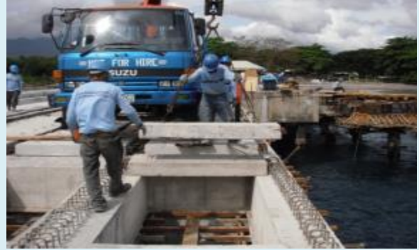
Setting pre-cast slabs on beams
